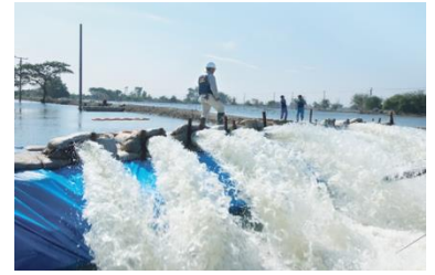
▲ Drainage works by the Japan Disaster Relief Team
