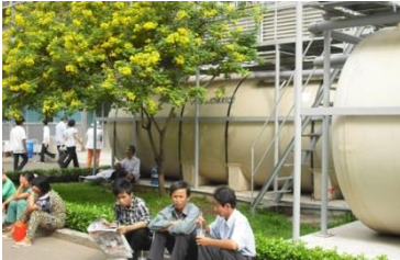
▲ Johkasou in hospital
