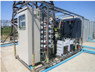
▲ Water treatment system introduced to Myanmar
