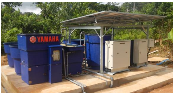
▲ Yamaha Clean Water Supply System
