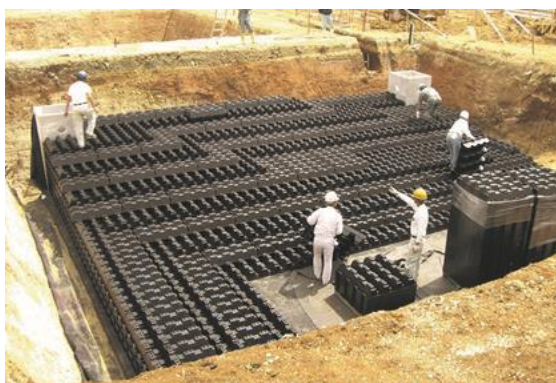
▲ Installation of CROSS-WAVE
