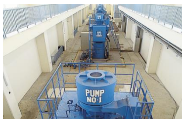
▲ Dual purpose pump station
